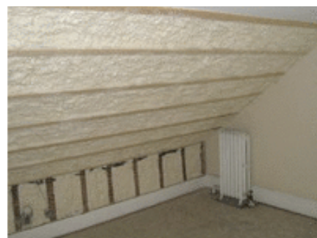
Use of spray foam insulation provided a tightly insulated attic
